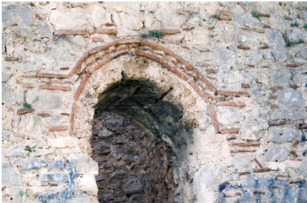
Fig. 49. Castle of Vonitsa, inner enceinte. Detail of masonry.
